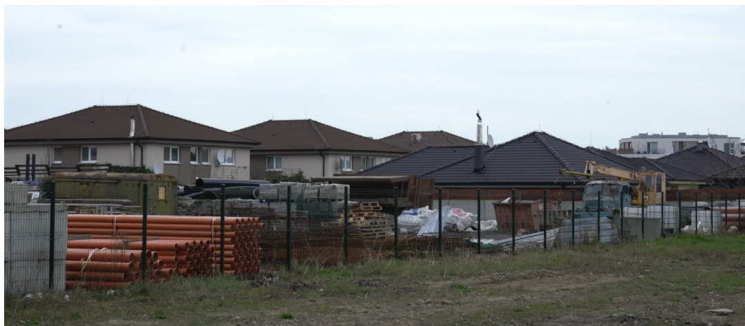
Fig. 2. Ongoing construction in Bratislava's suburban areas. Photo by Soňa G. Lutherová, 31. 3. 2023
